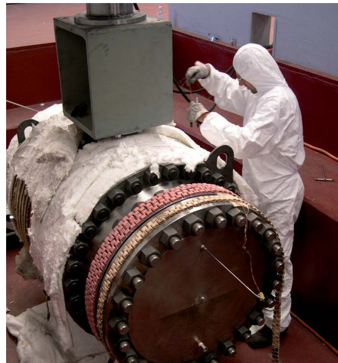
High Temperature Valve Testing
