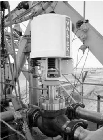
This cryogenic Mark One is used for aerospace testing as an O<sub>2</sub> vent.
