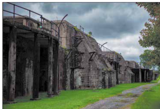
Behind the parapets, the earthen mounds into which were built the concrete bunkers.
