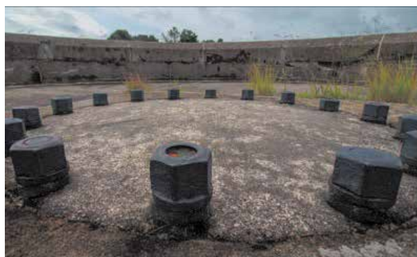
The nuts and bolts that anchored a 5-inch gun.
