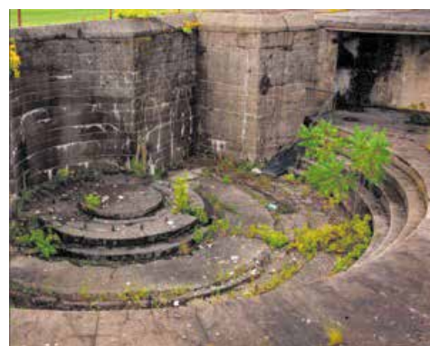
The remains of an emplacement for a 10-inc "disappearing gun, which could be quickly camouflaged after firing.
