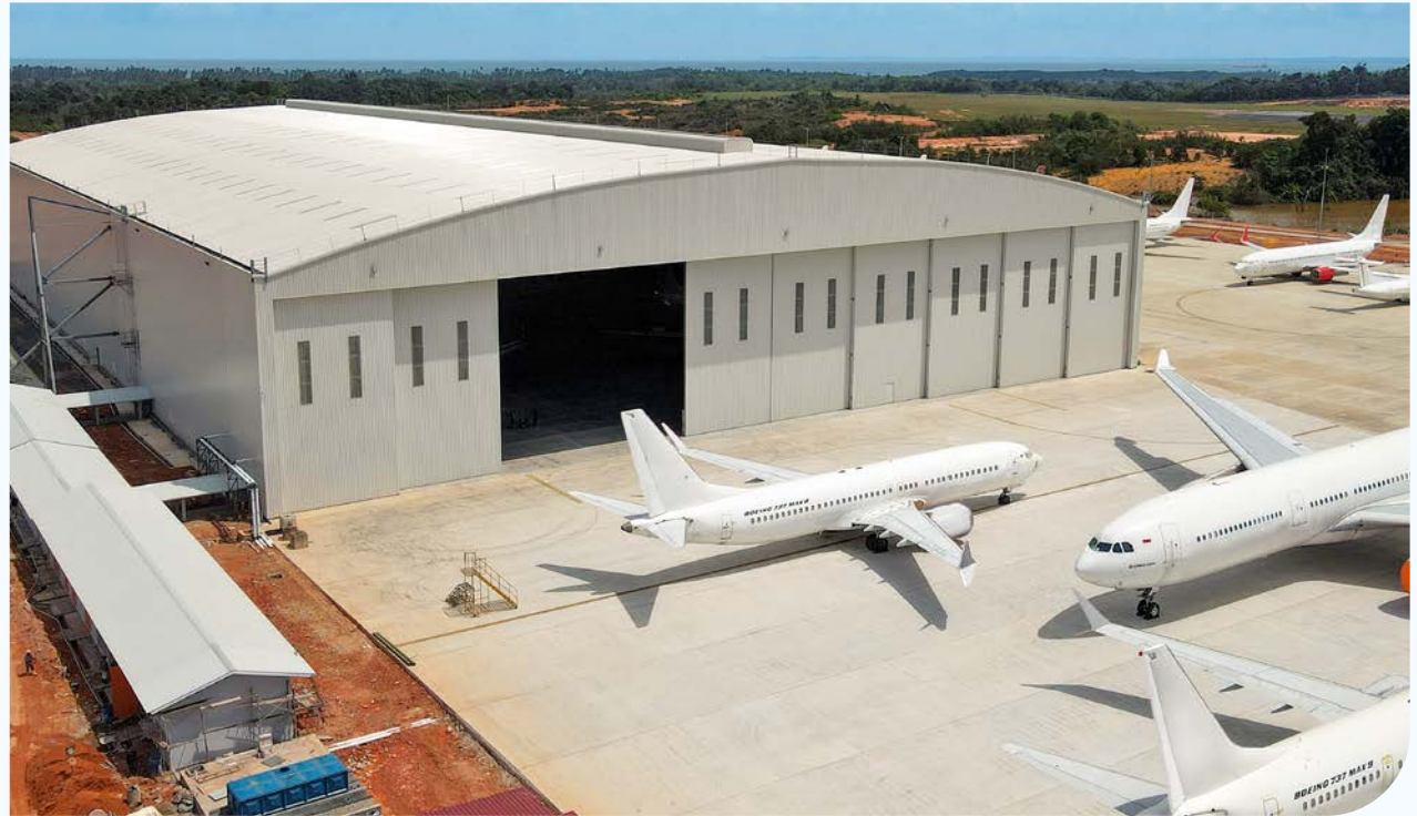
Hangar door and door track configuration for this project 5 tracks with 10 independent leaves (identical configuration on each end).
