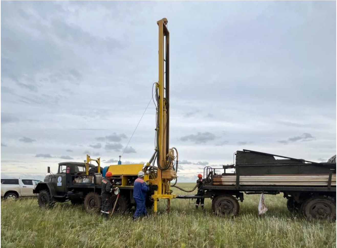
Figure 41: Burstroy KGK drill-rig.
