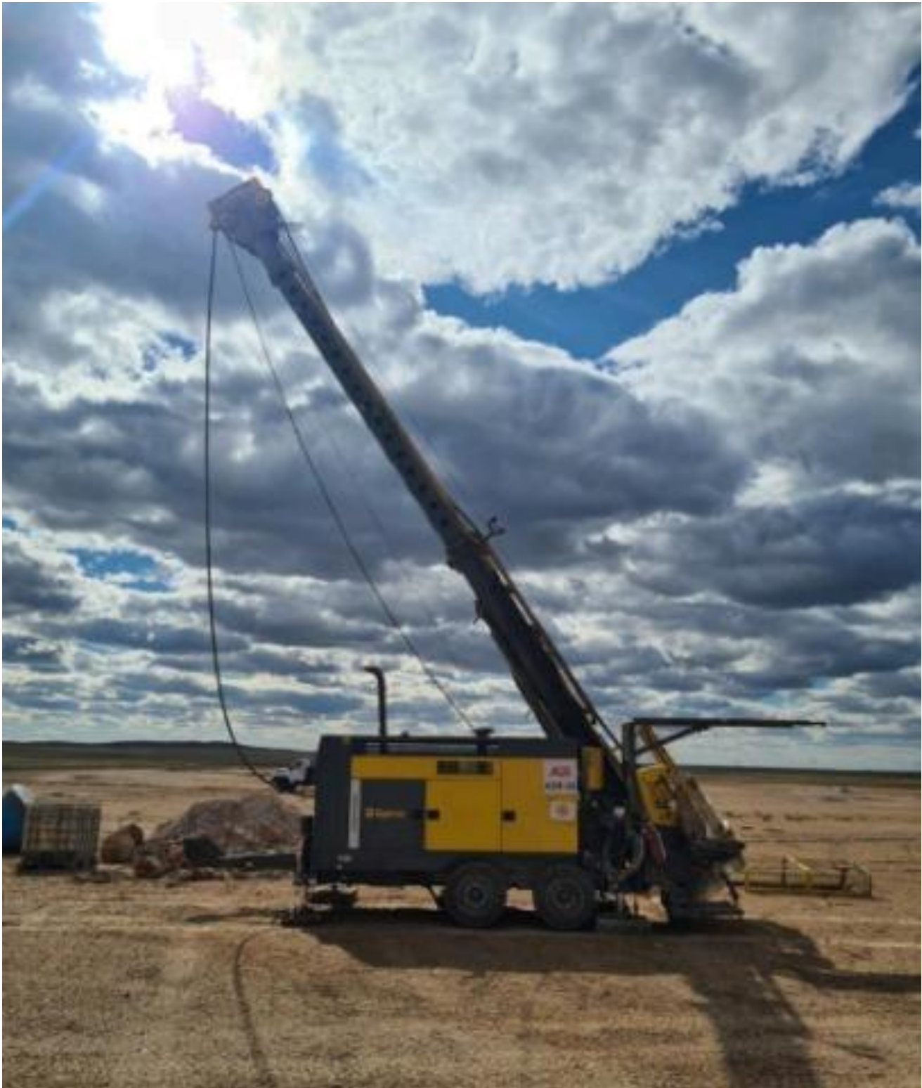
Figure 39: AQS Christensen 140 drill-rig
