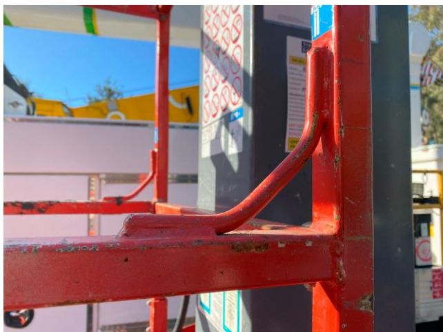
Photograph 3 – Lanyard Attachment Point
