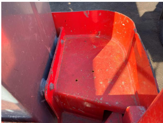
Photograph 5 – Typical General Frame Welds
