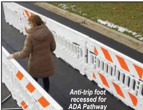
Create ADA Compliant Pedestrian Pathway
