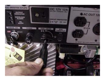
Disconnect battery cables. Then, remove 4 bolts that secure the front panel (2 on each side). Pull the front panel out and down.
