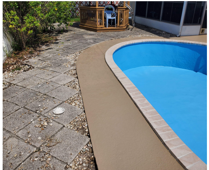
After application of Acrythane Concrete Stain
