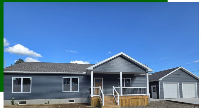
Photo (Above): The 14th home built through partnership with GST BOCES is having the finishing touches put on before getting ready to go out to bid. This home is on Canisteo Street. The project provides GST BOCES students with hands-on experience in residential construction while helping create new housing in the City.
