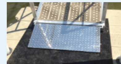
TRANSIT PLATE ENABLES EASIER ACCESS TO THE GANGWAY (WHEELCHAIRS, CARTS, ETC.).
