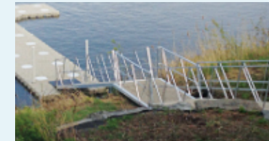
HANDRAIL INCREASES THE GANGWAY'S RIGIDITY AND SAFETY.
