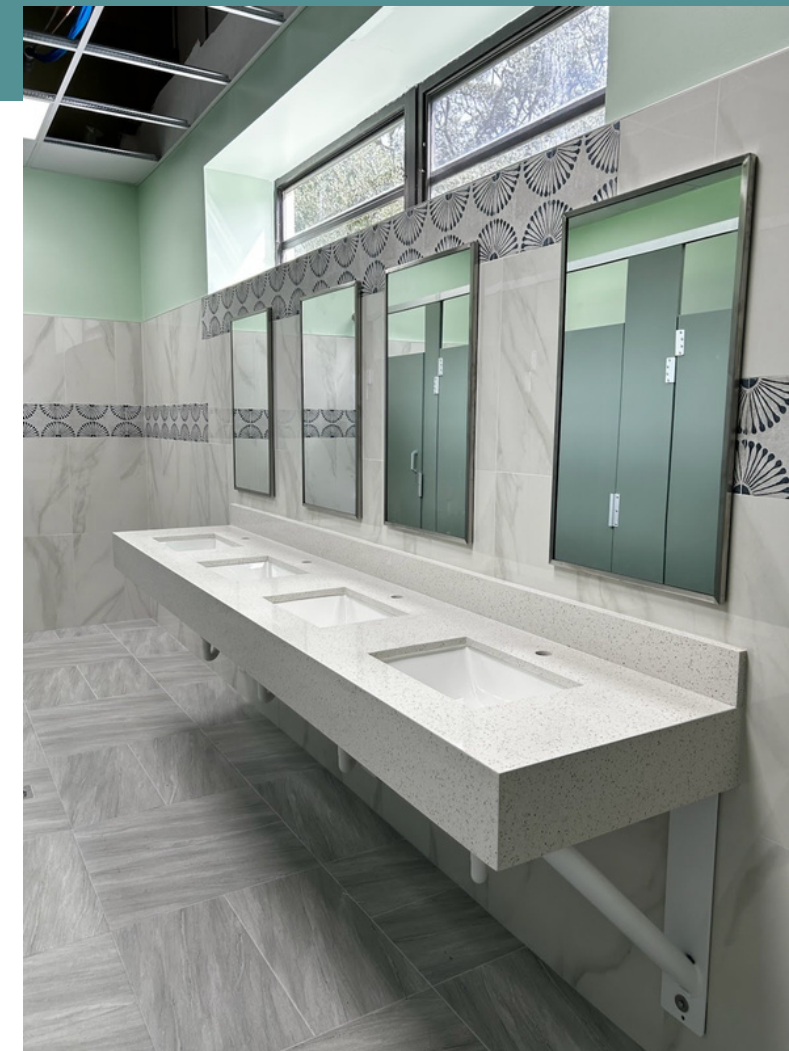
Renovated bathroom (middle view)
