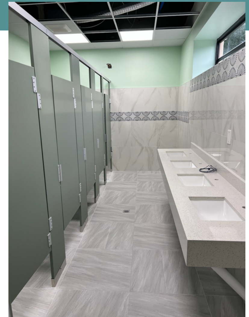
Renovated bathroom (front view)
