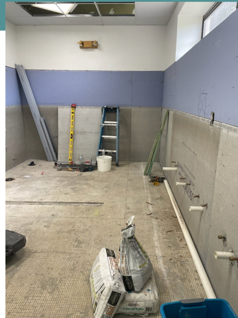
Demolition of bathroom
