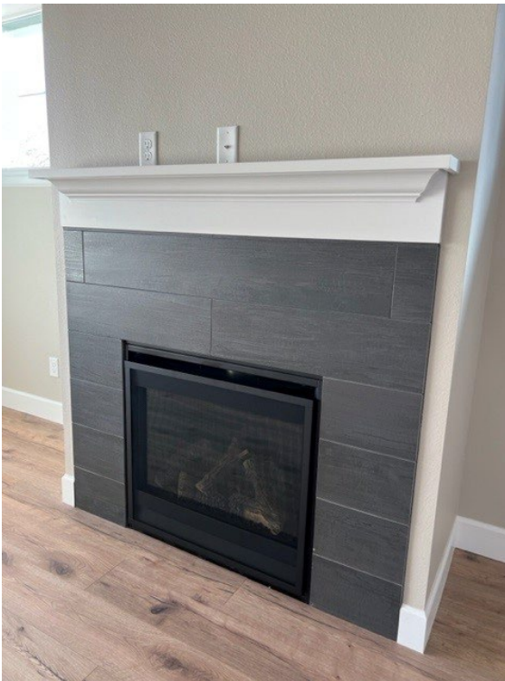
Standard - Gas Fireplace with Tile Surround
