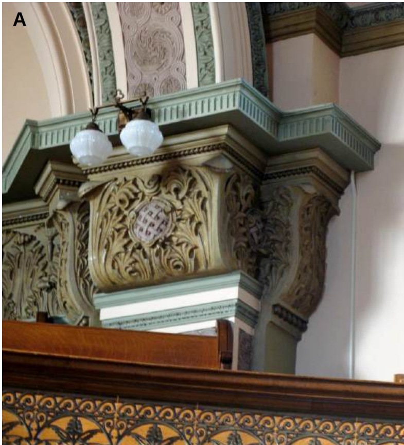
FIGURE 11. PILASTER (A) AT THE BASE OF AN ARMENIAN ARCH AND CORNICE MOULDING (B)
