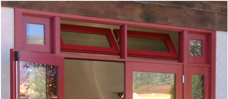
Standard Friction Hinged Mullied Transom Hoppers
