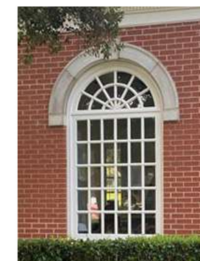
Half Circle Fixed Transom with Spoke TDL & Radius Bars muller above a Fixed Window
