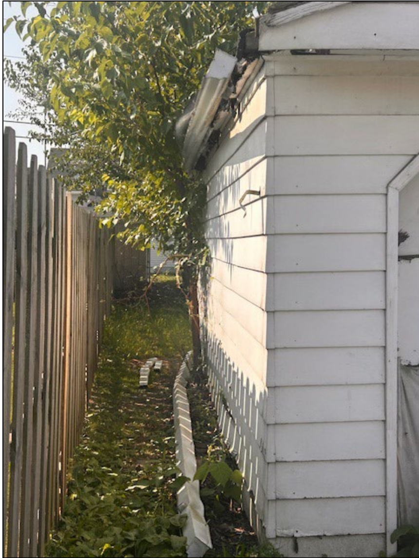
Photo 9: Garage, East Elevation, 23100 Ivan Avenue
