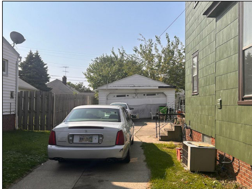
Photos 1 and 2: Single-Family Home in Foreground, with Garage in Background; North Elevation of Garage, 23100 Ivan Avenue
