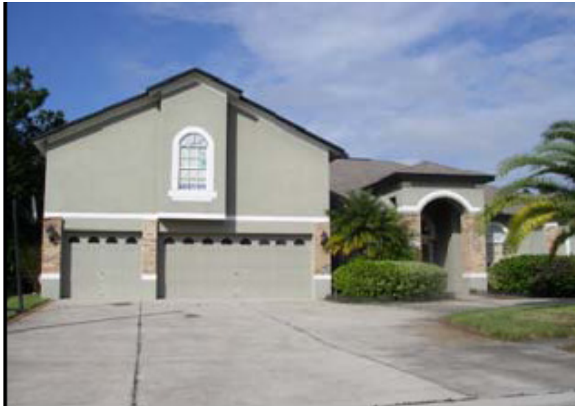
Unacceptable: "lopsided" upper floor on one side.
