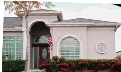
Unacceptable: plastic panels permanently attached to home.
