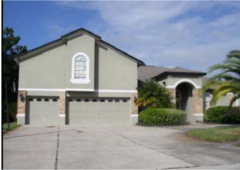
Unacceptable: "lopsided" upper floor on one side.
