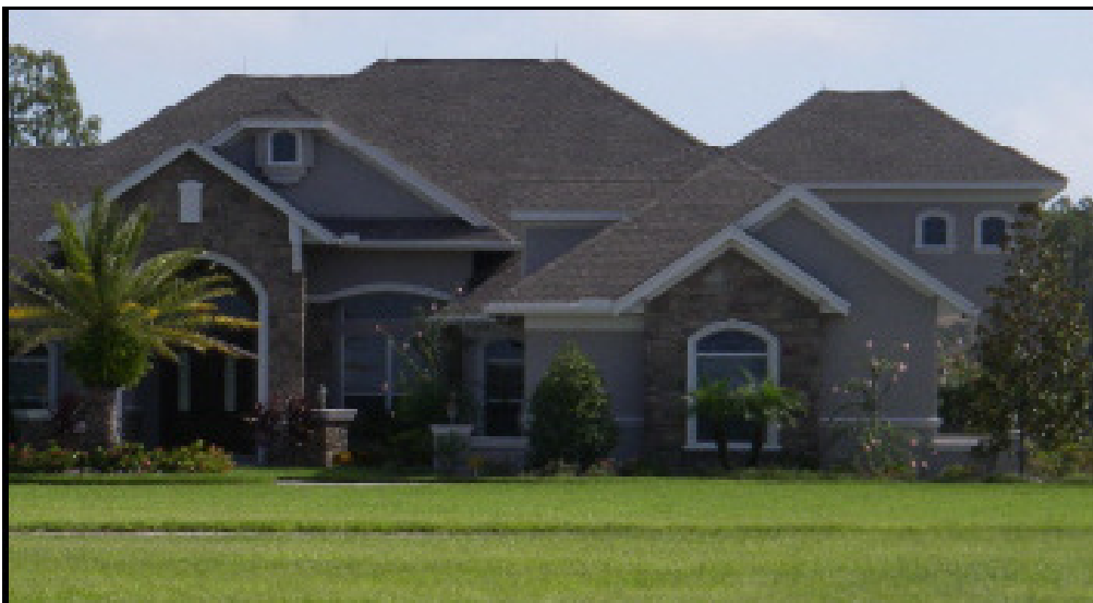
Acceptable: upper floor placed at rear of one story home.
