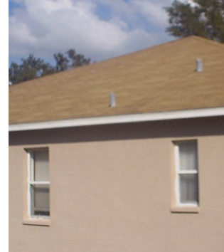
Unacceptable: unpainted flashing and roof drip edge
