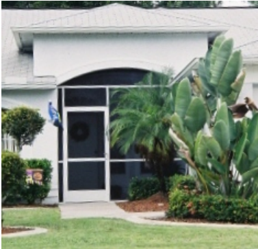
Unacceptable: screened in front porch
