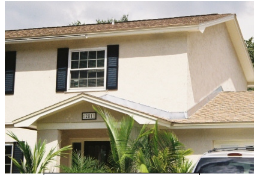
Unacceptable: unpainted flashing and roof drip edge
