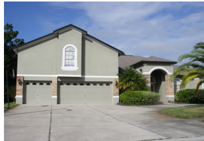
Unacceptable: “lopsided” upper floor on one side
