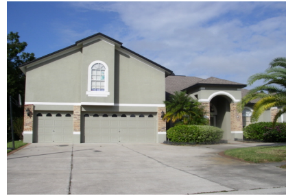
Unacceptable: “lopsided” upper floor on one side
