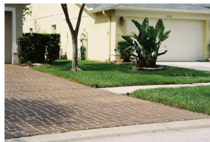
Unacceptable installation: paver material not flush with curb and street sidewalk. The paver material itself is acceptable.
