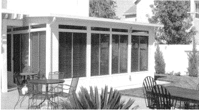
Unacceptable: Flat roof sunroom
