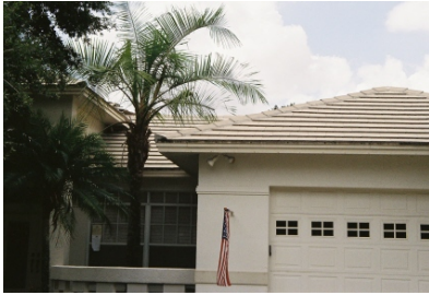
Acceptable: flat tile roofing
