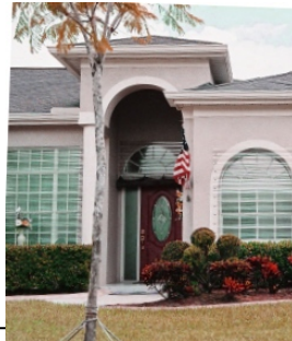
Unacceptable: plastic panels permanently attached to home.
