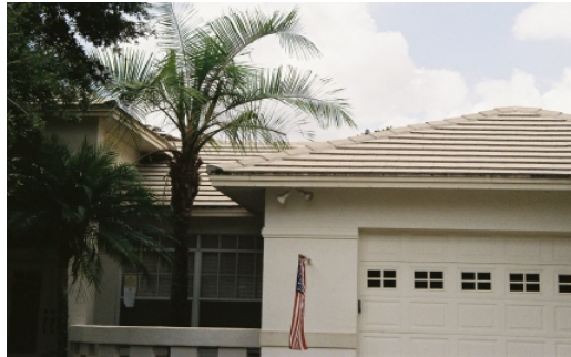
Acceptable: flat tile roofing
