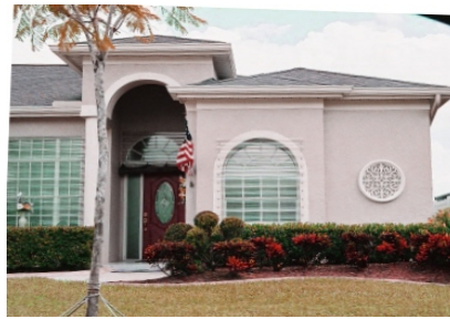
Unacceptable: plastic panels permanently attached to home.
