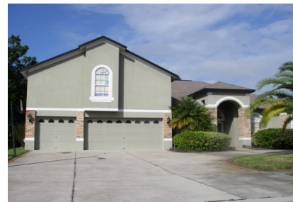
Unacceptable: “lopsided” upper floor on one side
