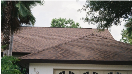
Acceptable: Minimum 30-year asphalt dimensional shingle
