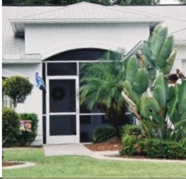
Unacceptable: screened in front porch
