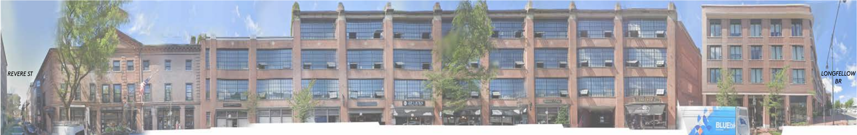
CHARLES STREET WEST ELEVATION – LARGER OPENINGS / PIERS WITH ORNATE AND NON-TRADITIONAL BRICK MASONRY
