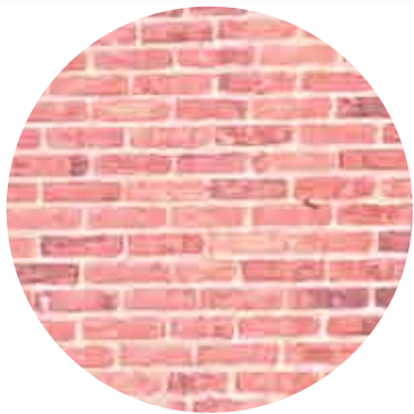
TRADITIONAL RUNNING BOND MODULAR BRICK (142-162 Charles St)
