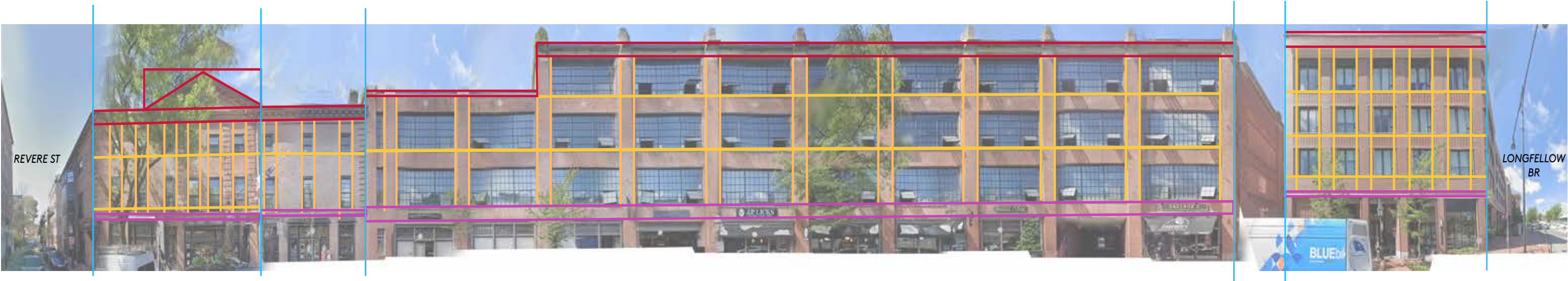
CHARLES STREET WEST ELEVATION – LARGER OPENINGS / PIERS WITH ORNATE AND NON-TRADITIONAL BRICK MASONRY
