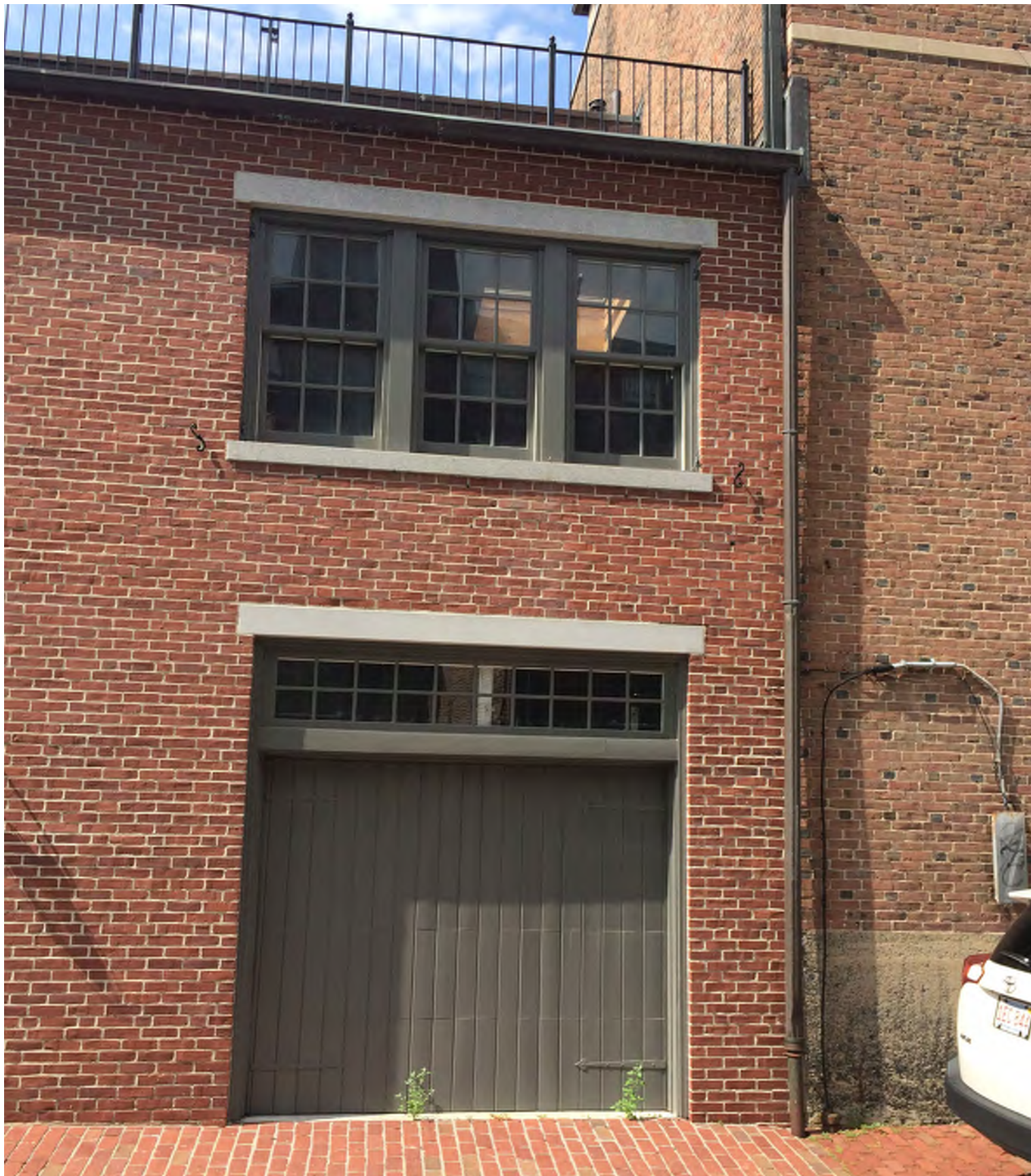
1. VIEW OF GARAGE
