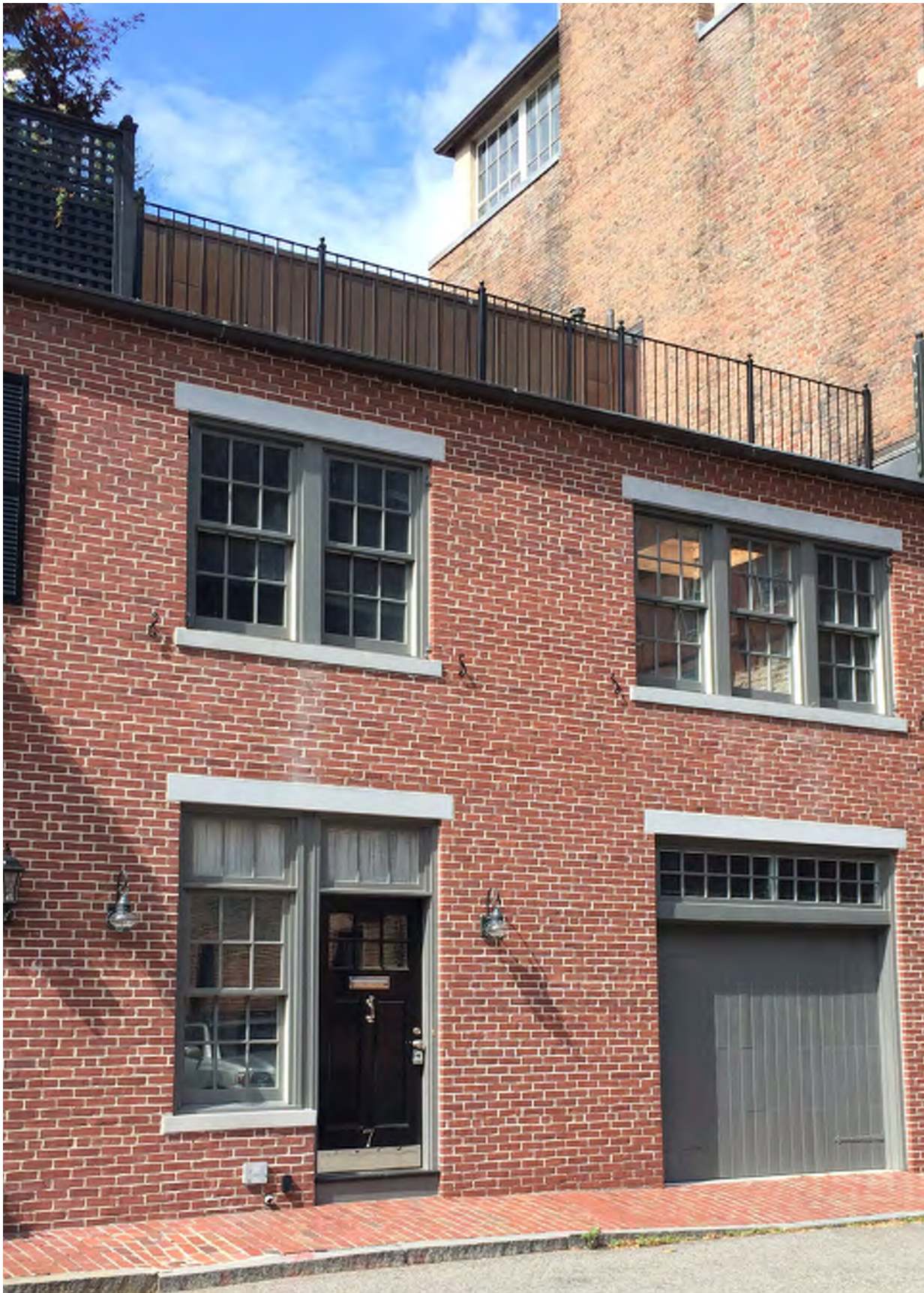
2. VIEW FROM WEST
