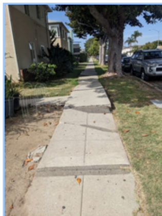
Sawtelle Sidewalk Improvement Project - Before
