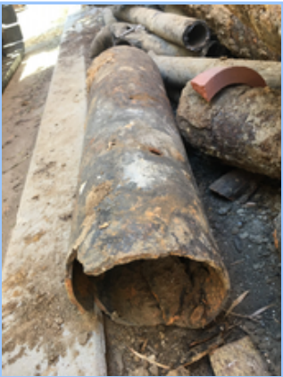
Emergency sewer repair
