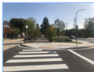
Culver Boulevard Pedestrian and Bike Safety
