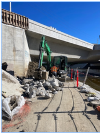
Higuera Bridge maintenance
