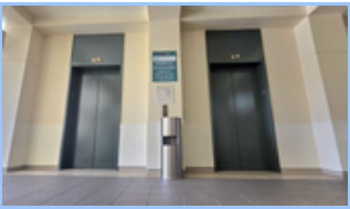
City Hall passenger elevators
