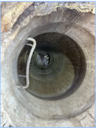
Existing 57-inch concrete pipe and manhole
