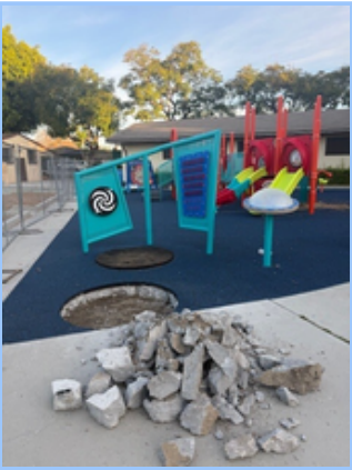
Citywide Park Playground Repairs
