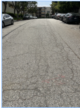
Pavement Rehabilitation - Before
