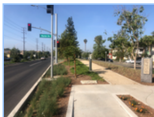
Culver Boulevard Pedestrian and Bike Safety
