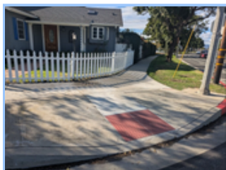
Sawtelle Sidewalk Improvement Project - After
