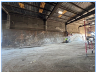
Construction of Transfer Station push wall
