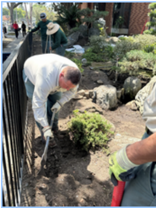
Park Irrigation System Maintenance / Upgrades
