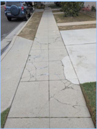
Before sidewalk repairs
