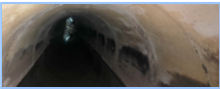
Existing 57-inch concrete pipe and manhole
