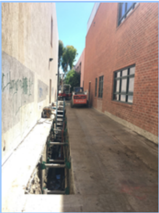
Emergency sewer repair
