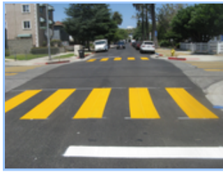
Pavement Rehabilitation project
