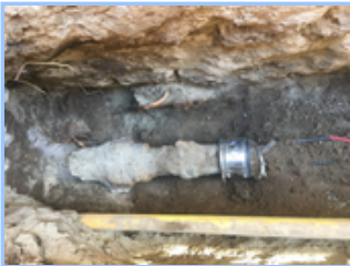
Emergency sewer repair
