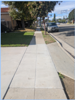
After sidewalk repairs
