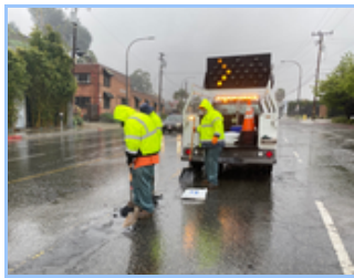
Pot hole repair
