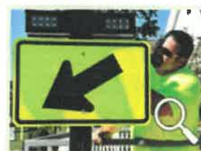
Bryan Lloyd installing sign
