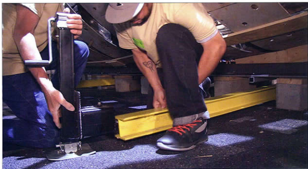
Loading cross member lifting jacks under La Bell support structure
