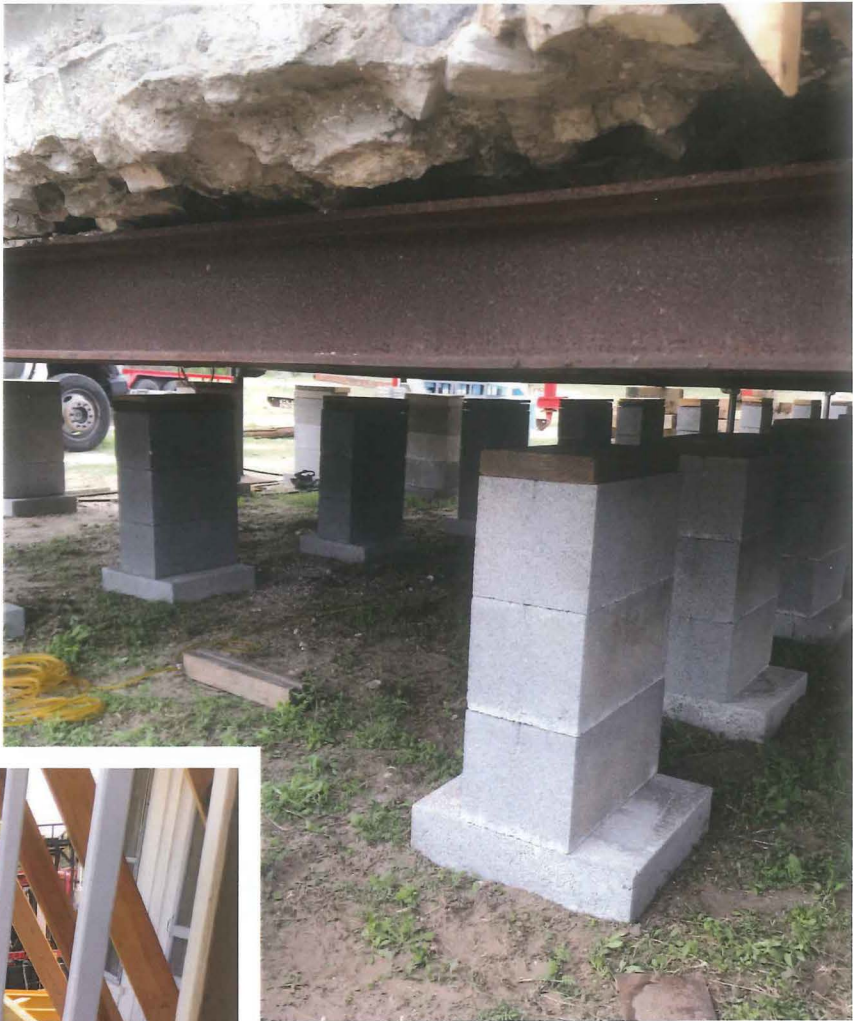
Ready to lower onto the new piers.
