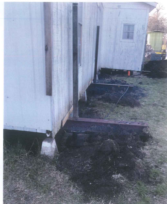
Cross-loaders installed, using our tall stacks that we use all the time.
