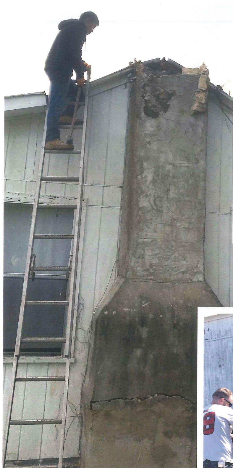
Disassembling the chimney.
