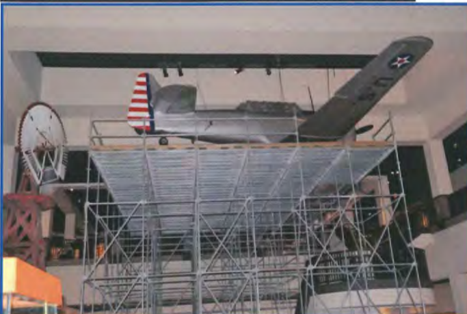
View of scaffold with aircraft lifted off the floor surface.
