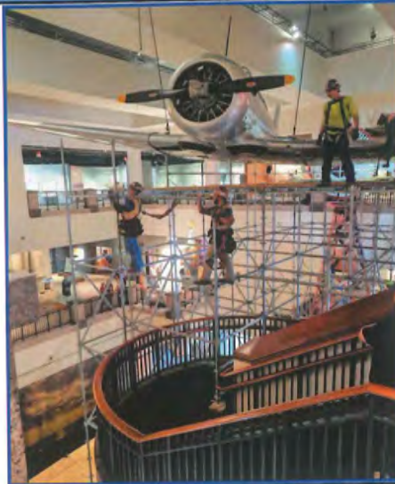
Scaffolding tear down in process; aircraft fully suspended.
