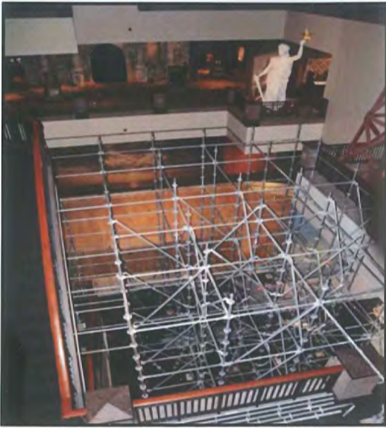
Almost to 3 rd floor. "Dance floor" in place ready for the Texan's move.
