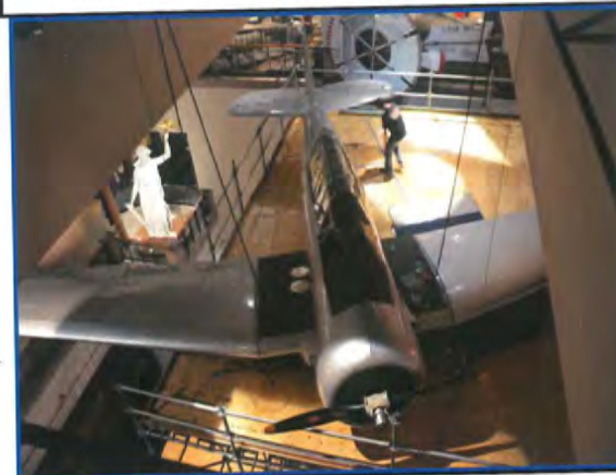
Primary cables rigged in place. Getting ready for the tail plane
