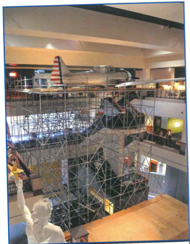
Ready for the rigging process
