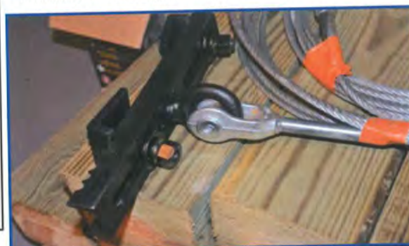
Main beam clamps with cable ready to install
