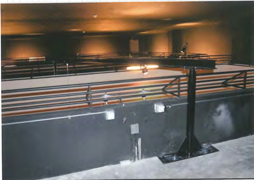
Re-located gantry beam in place, spanning the atrium
