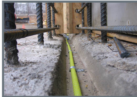
Figure 5. Anchoring clips on Injecto.
