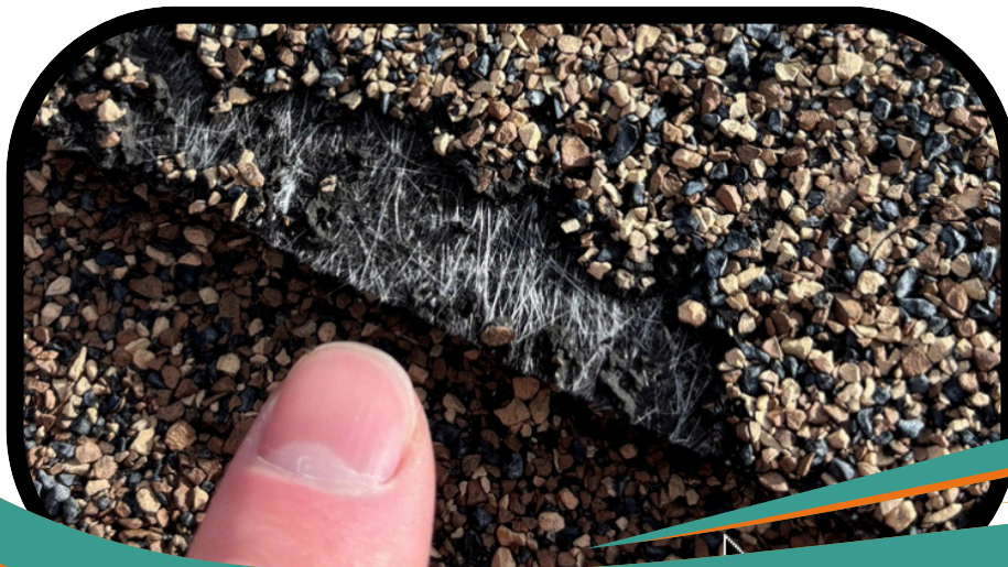
Exposed Fiberglass
