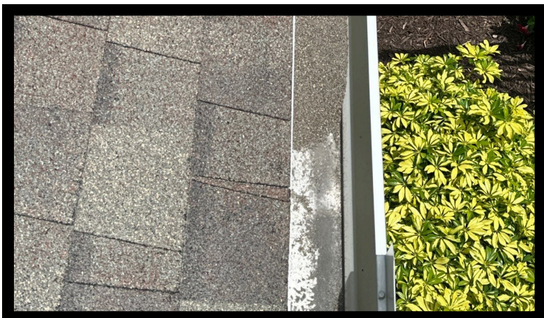
Granules in the Gutters
