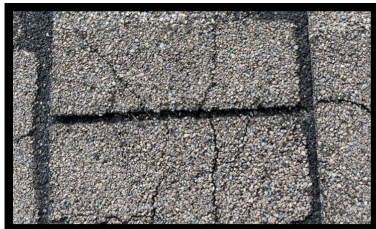
Cracking or Splitting
