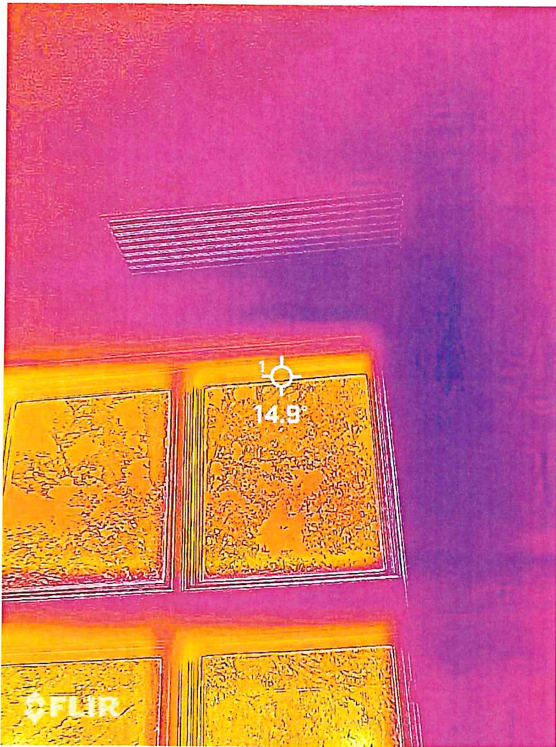
29 45-East Inside 1 above window Date Taken: 6/18/2026
