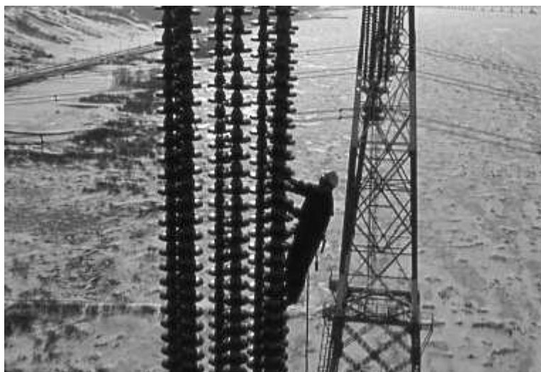
Final inspection by Michel Bornais of a 735kV suspension insulator on a tower over the St. Lawrence River, spring 1966, near the village of St-Laurent, Ile d'Orléans. (Collection of Michel Bornais)
