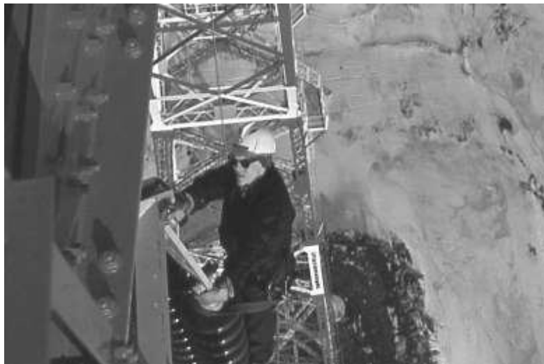
Final inspection by Michel Bornais of a 735kV suspension insulator on a tower over the St. Lawrence River, spring 1966, near the village of St-Laurent, Ile d'Orléans. (Collection of Michel Bornais)
