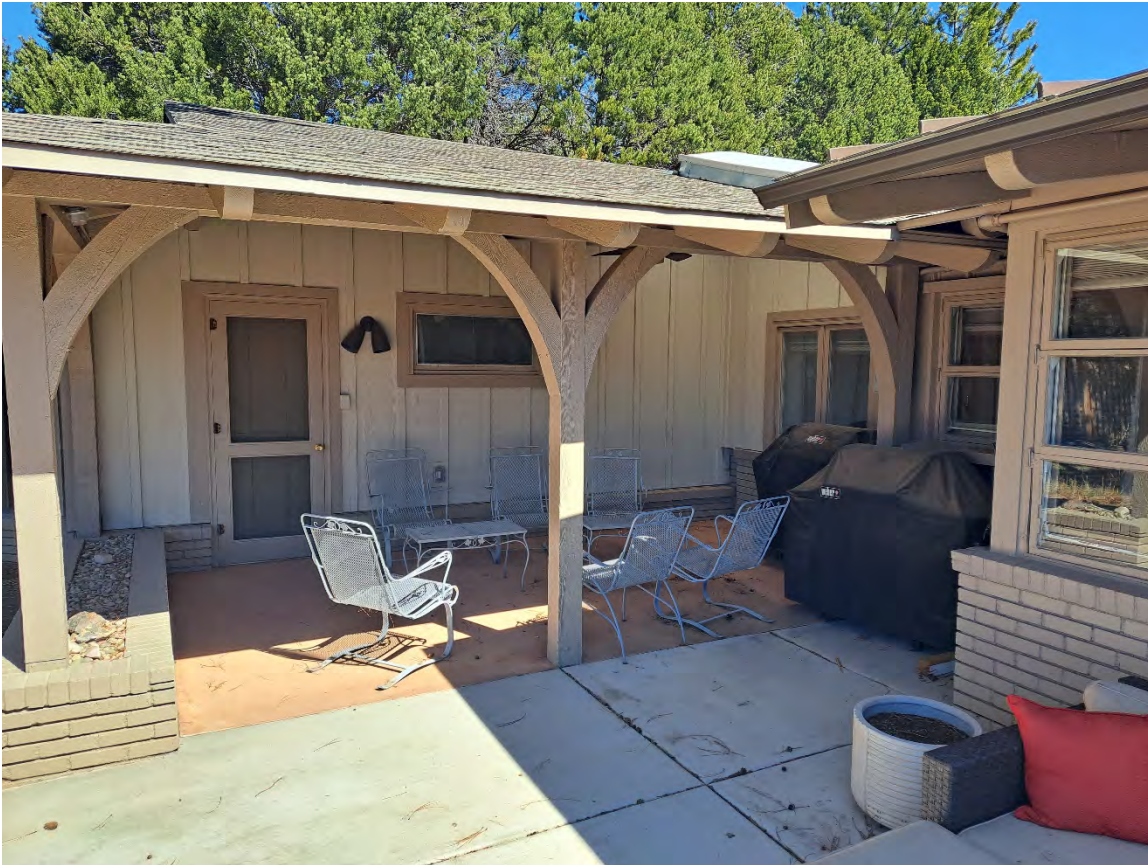
Photo 22: Facing North, South elevation of covered patio
