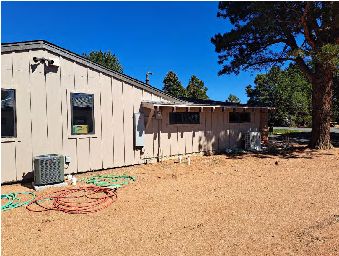
Photo 31: Facing North, South elevation
