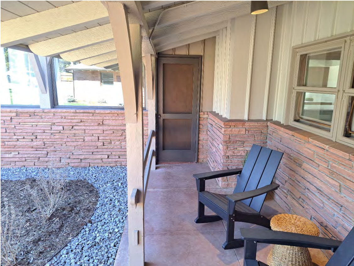
Photo 4: Facing South, Entry to offices
