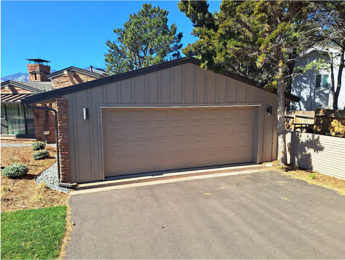
Photo 13: Facing Southwest, Garage
