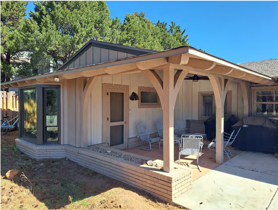
Photo 21: Facing Northeast, Covered patio
