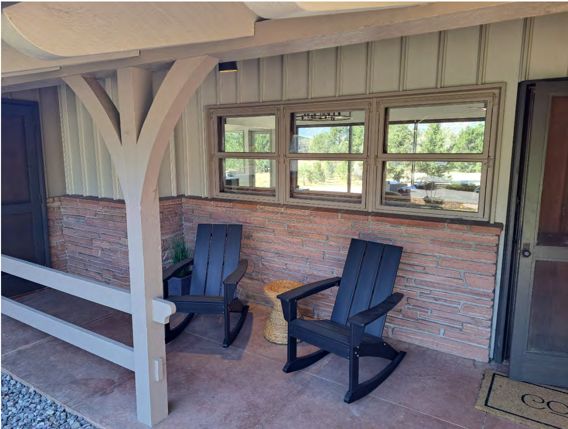
Photo 5: Facing West, Close up of windows to living room
