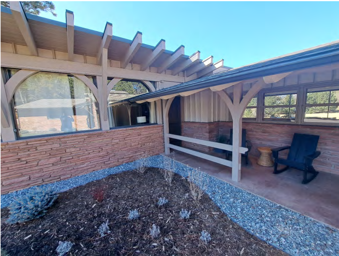
Photo 3: Facing Southwest, East elevation/Offices
