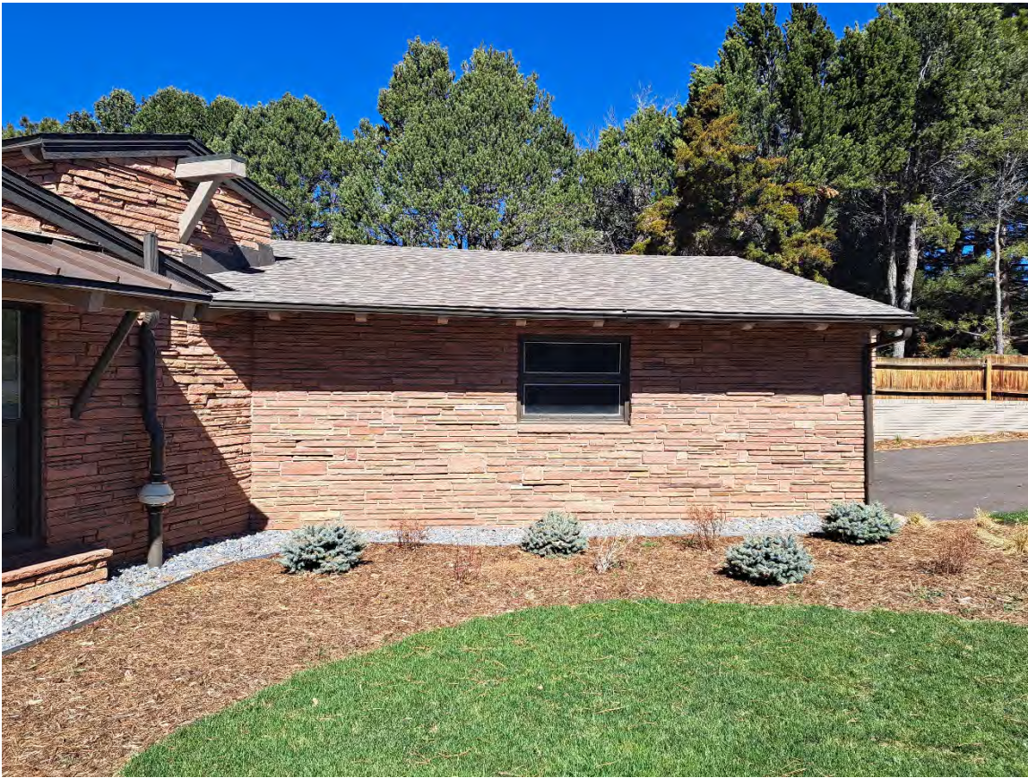
Photo 11: Facing North, South side of garage
