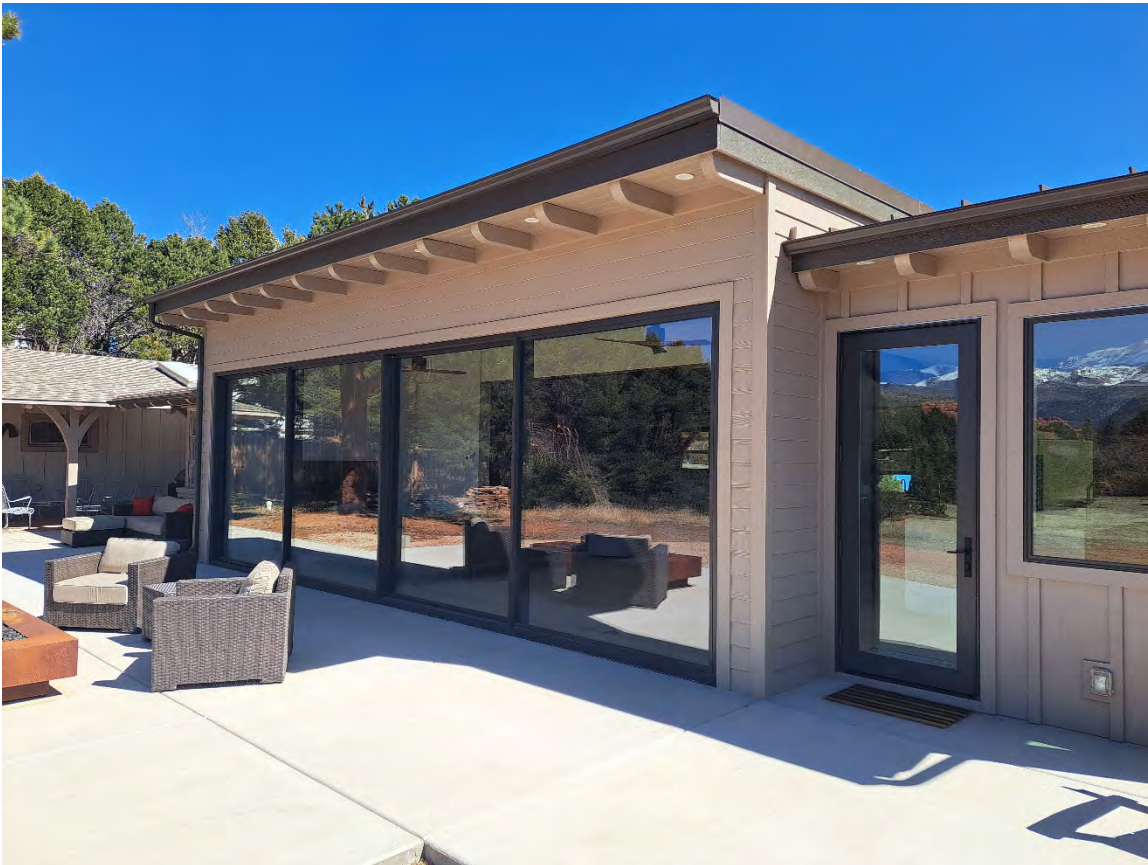
Photo 27: Facing Northeast, West elevation
