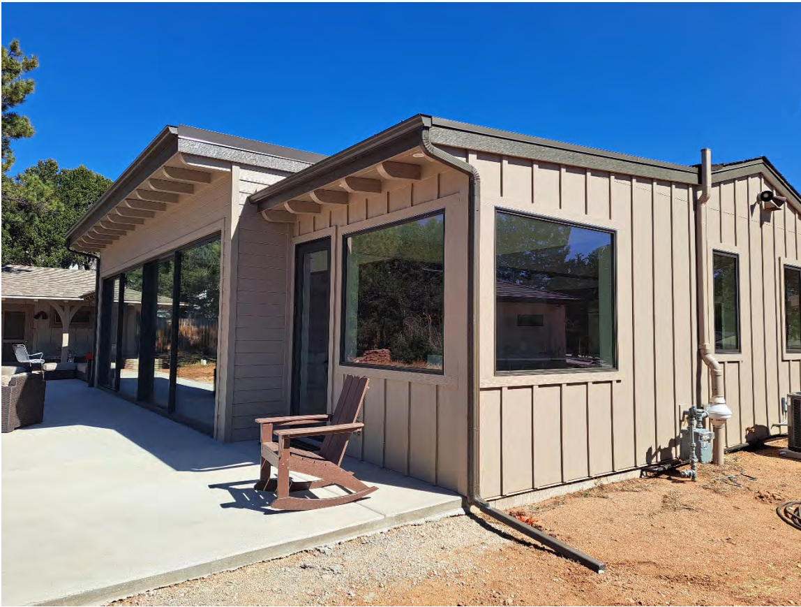
Photo 29: Facing Northeast, Southwest elevation
