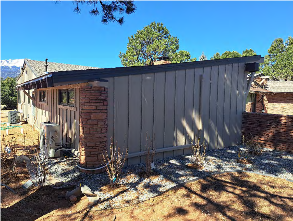
Photo 32: Facing West, East elevation
