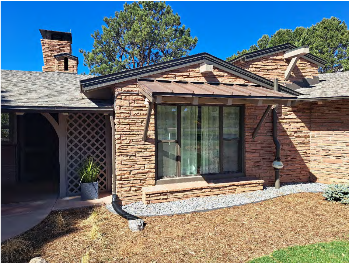
Photo 9: Facing West, East elevation
