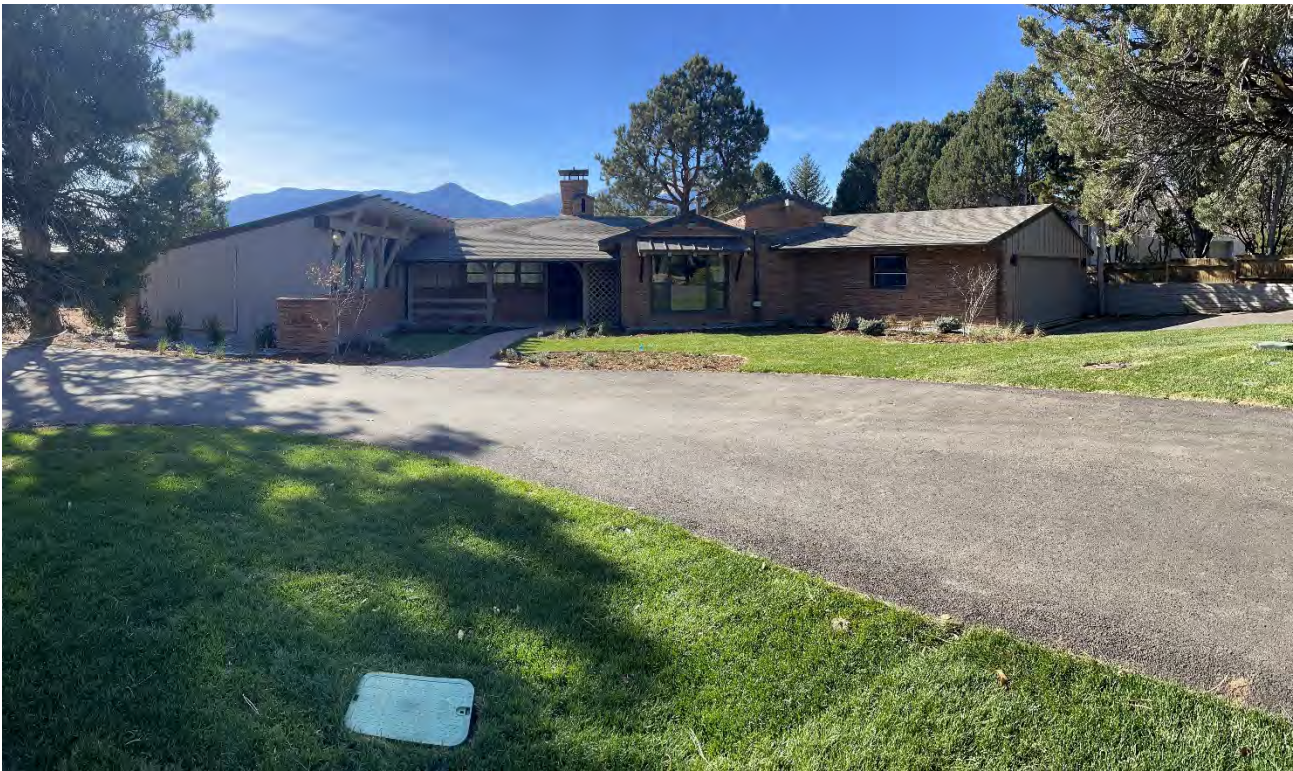
Photo 1: Facing West, East elevation
