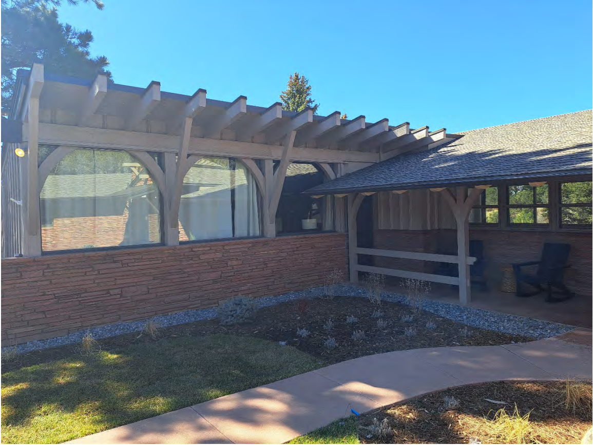
Photo2: Facing Southwest, East elevation/Offices
