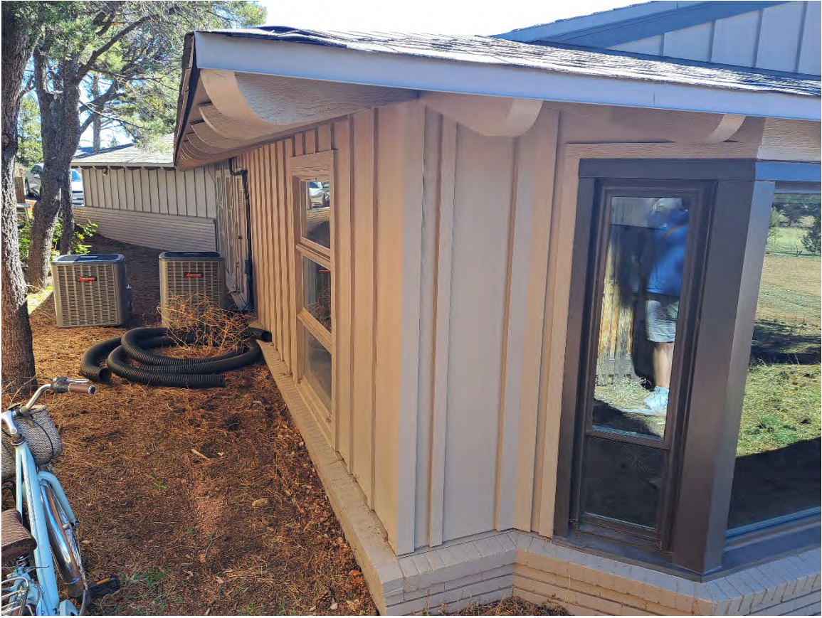
Photo 17: Facing Southeast, Northwest elevation
