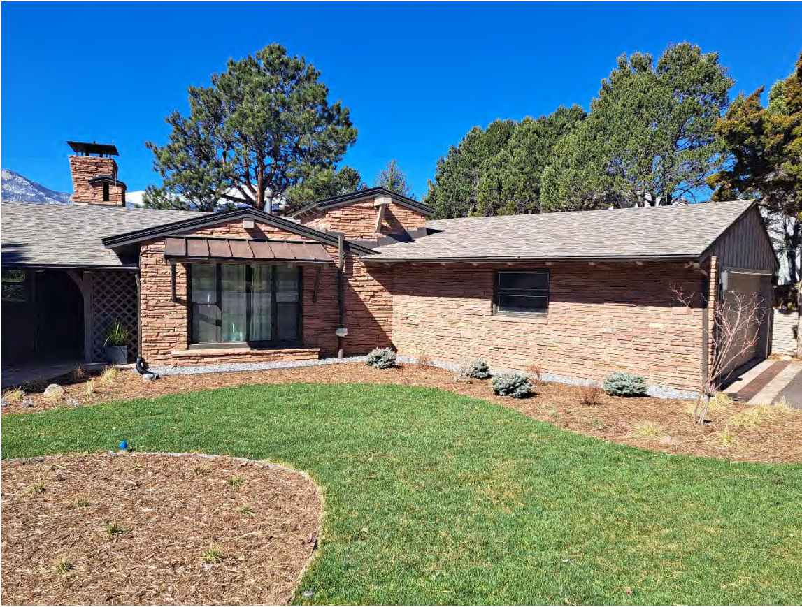
Photo 12: Facing West, East elevation
