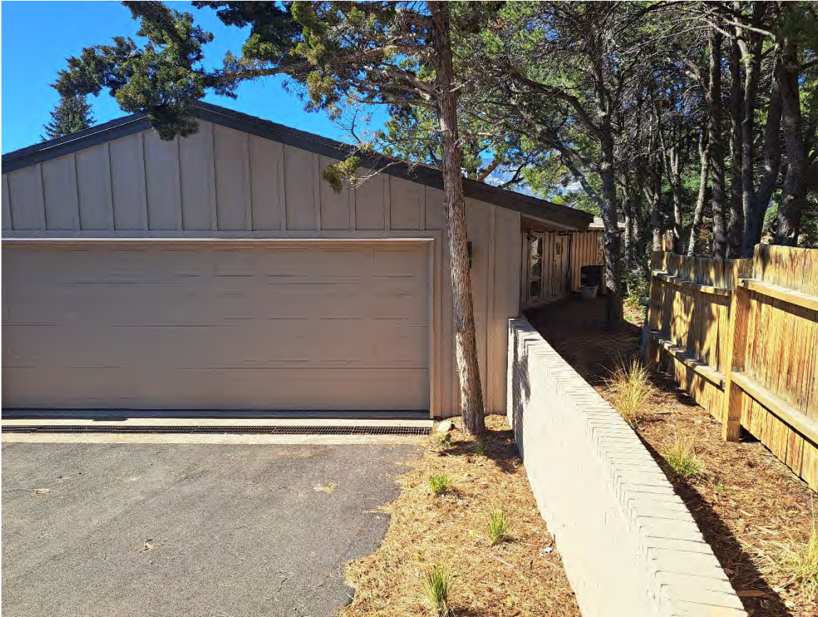
Photo 14: Facing West, Garage and North elevation
