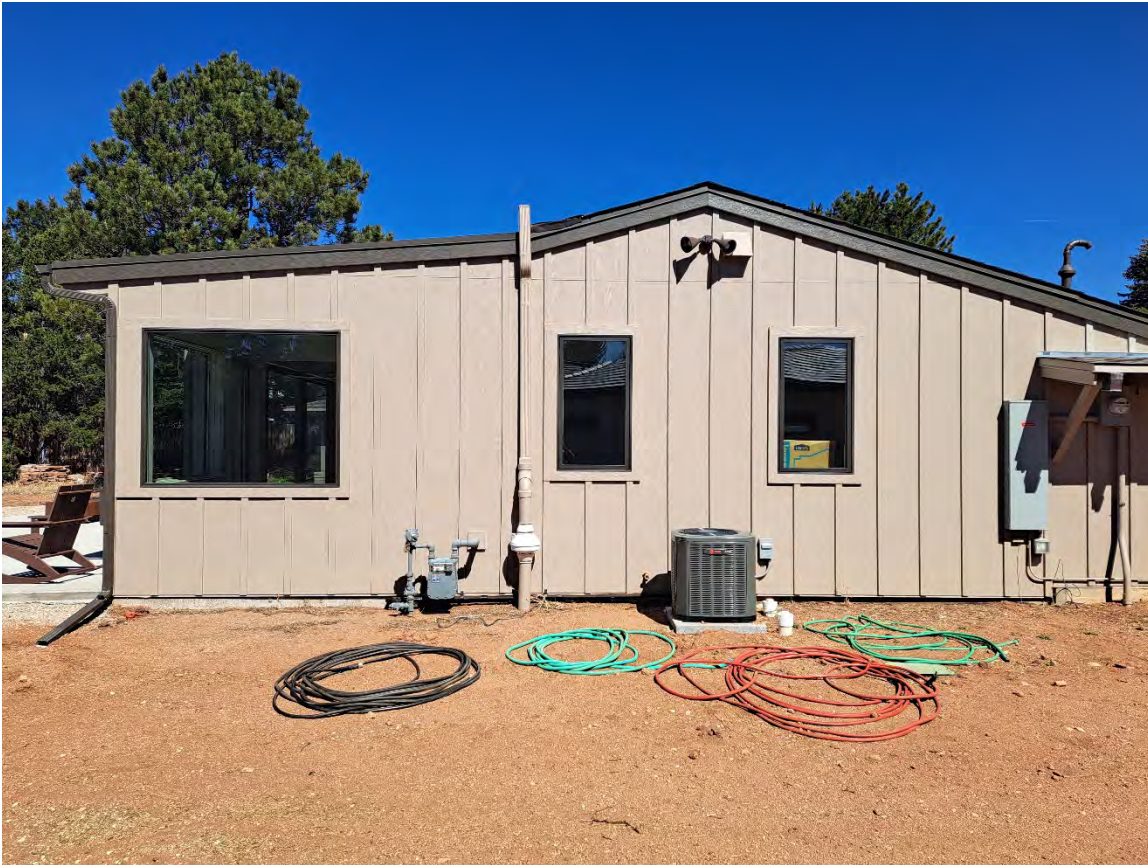
Photo 30: Facing North, South elevation
