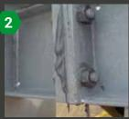
Connect components and remove excess MM1018.
