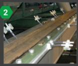
Injection points have been placed and MM1018 FL has been injected.
