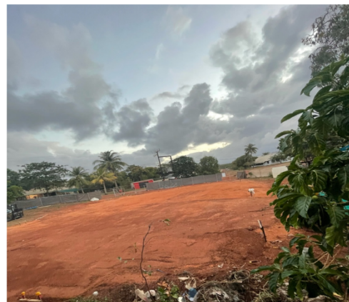
New Aged Care building under construction.
