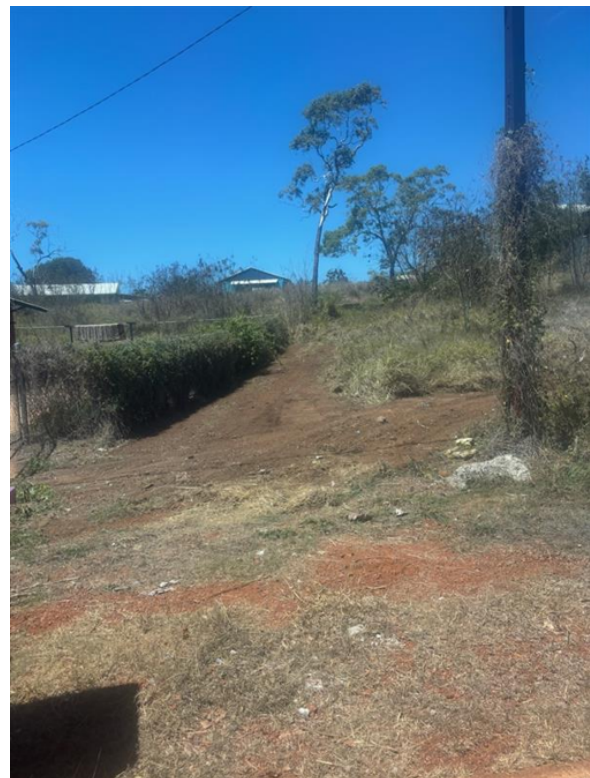
Drainage cleaning works
