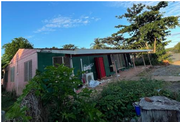
Old Aged Care Building
