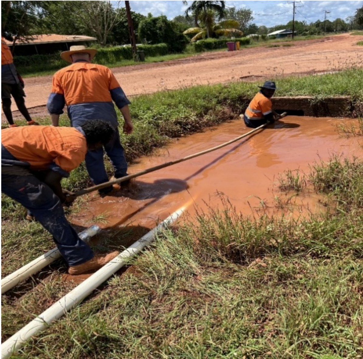
MS team working on clearing drainage.
