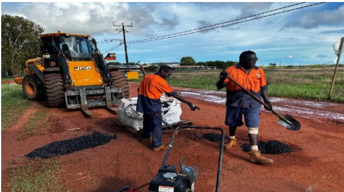
Figure 3. MS team members, Daniel & Neil sealing potholes before the next rain.
