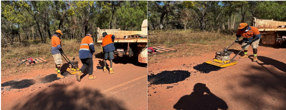
Municipal Services (MS) team repairing potholes on Airport Road
