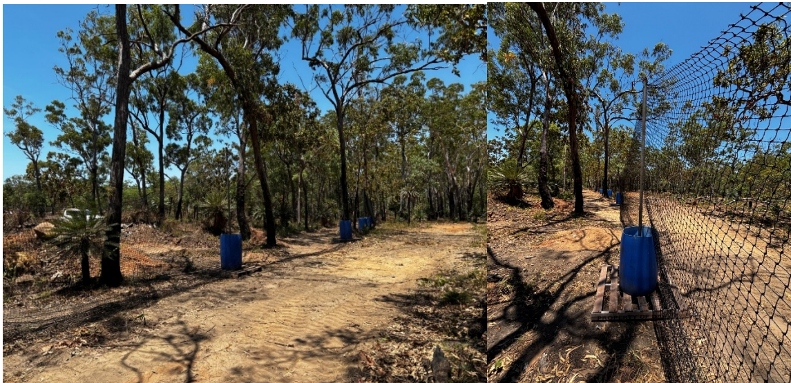
New netting installed at the landfill.
