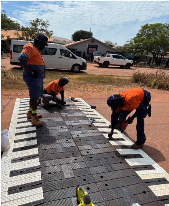
New speed bump installation.
