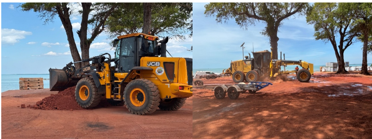
MS team and External stakeholders working together in grading the barge landing area.
