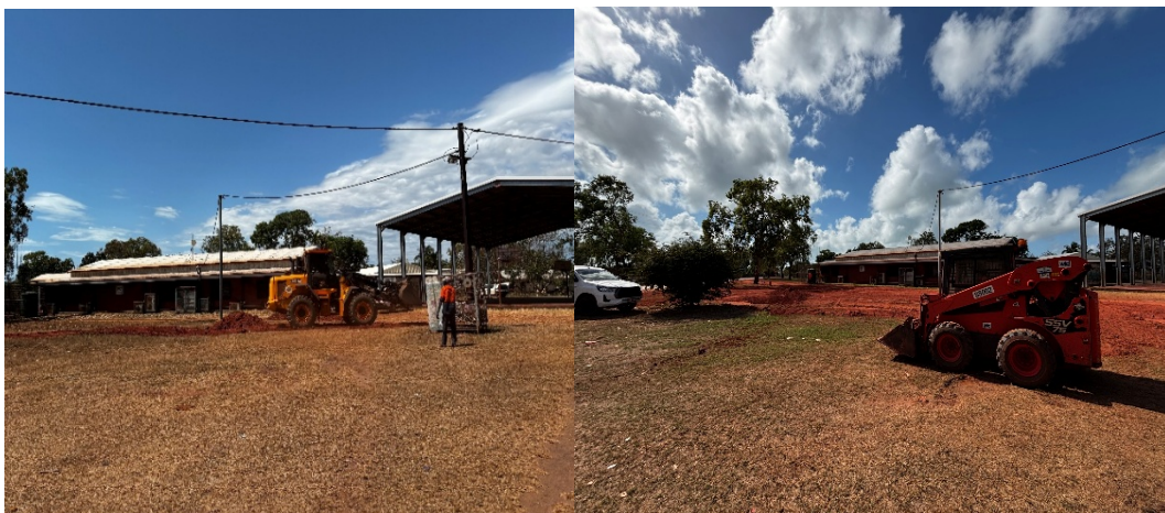
MS team and WTD working together at Rec Hall area using lots of gravel
