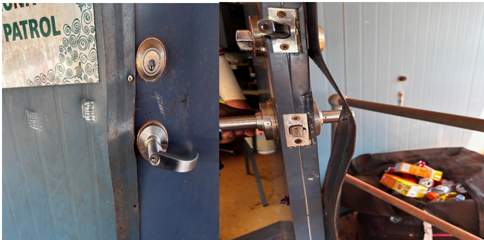
The Office door pried open and deadbolt damaged using a heavy tool
