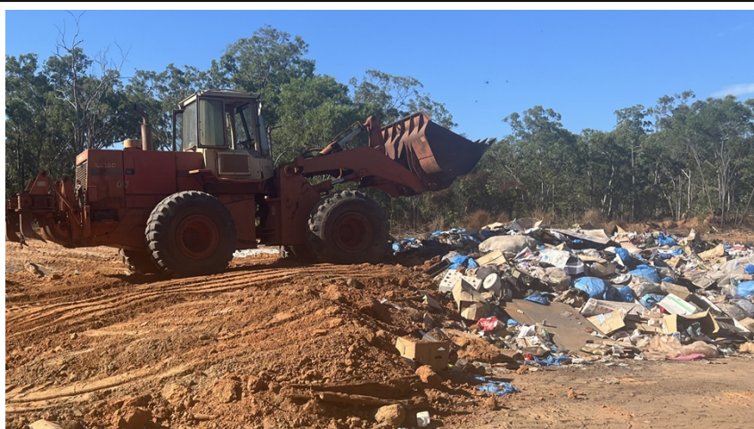
Capping General Waste
