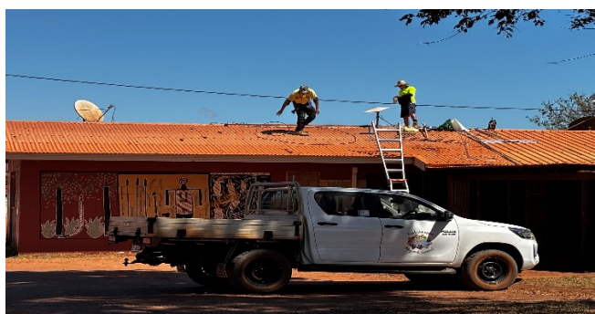
TEABBA team installing the hardware
