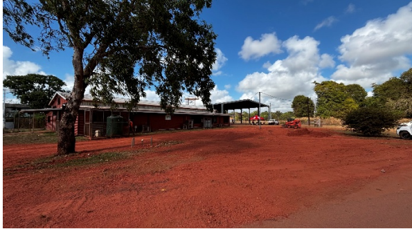
EARC Rec area after works have taken place
