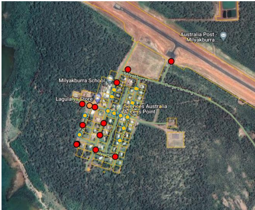
Figure 1 Streetlights identified as not working.
