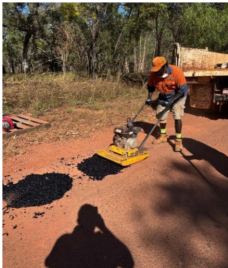
Pothole repairs
