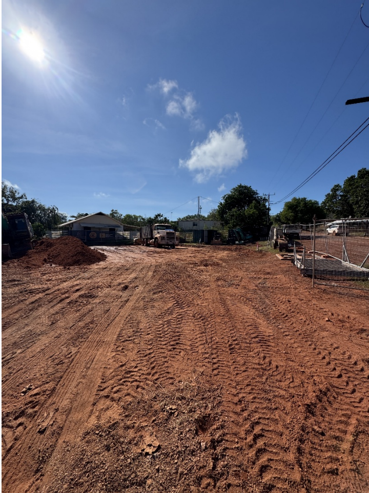
Image – Existing Aged Care Centre demolished, and area prepped for new build
