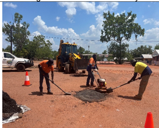
Gapuwiyak MS team repairing potholes
