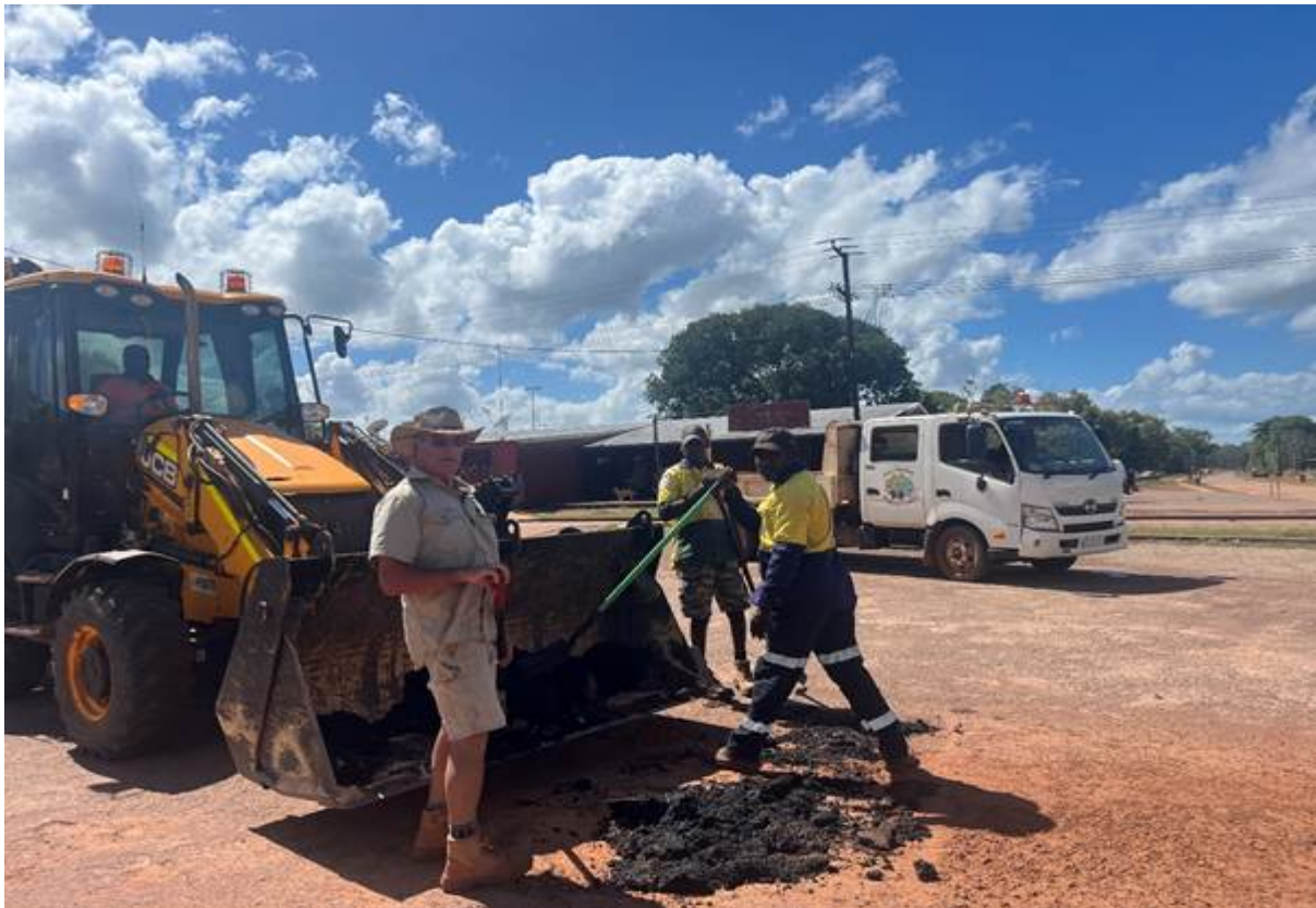
Another day, another pothole patched! Keeping our roads safe and smooth.
