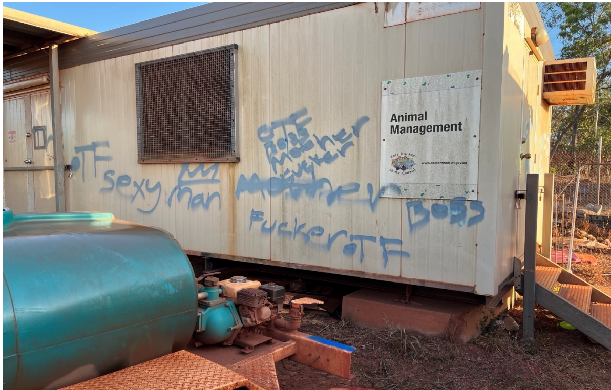
Animal Management building in Municipal Services yard
