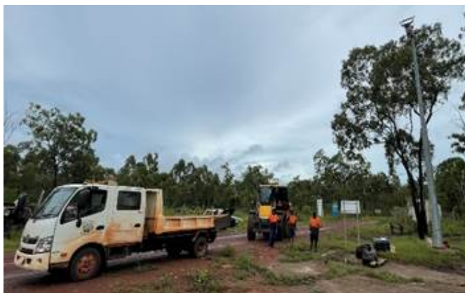
Galiwinku Municipal Services assist in CCTV installation
