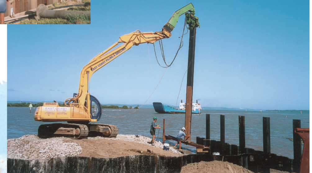
Right: Construction of a Barge Berthing Dock at Toondah Harbour, Cleveland.
