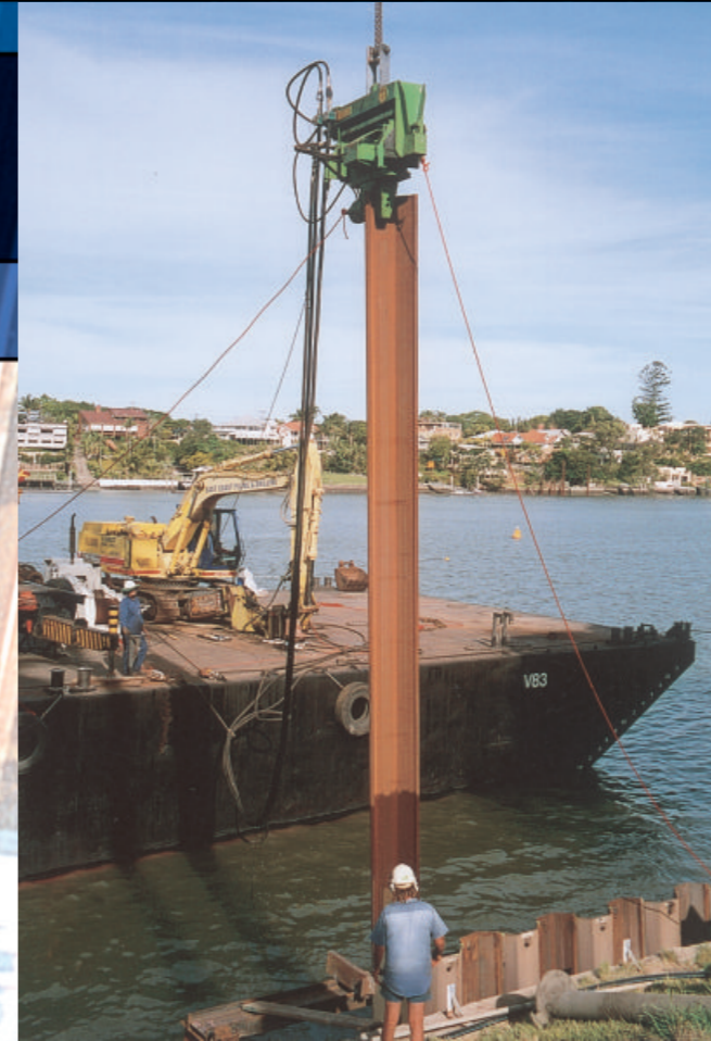
Above: Revetment wall construction at New Farm on the Brisbane River.
