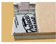
Water Penetration Barrier Below Each Window and Mullion with Sill Pan.
