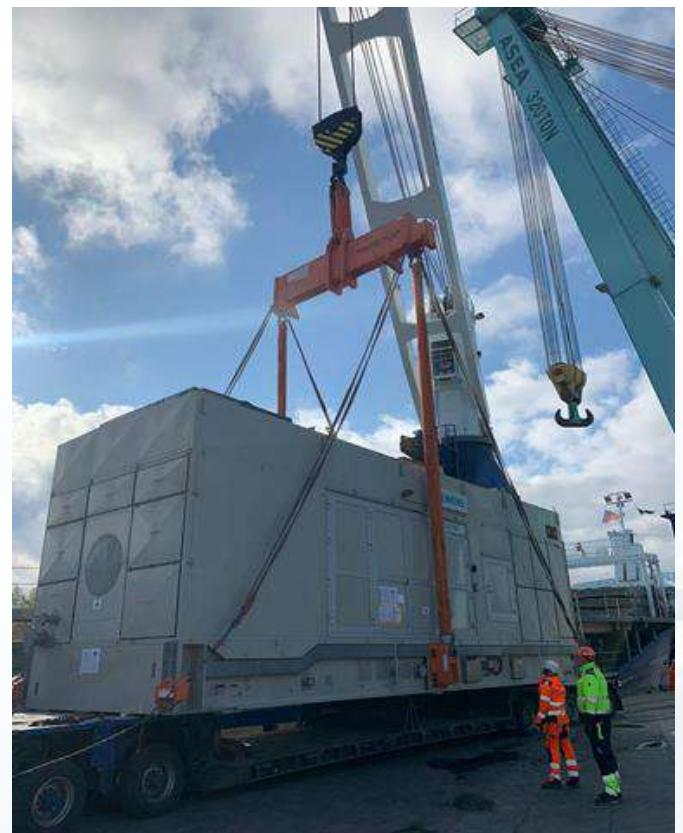
**Transformer - Weight(128 Ton) From: Italy To: Spain**
